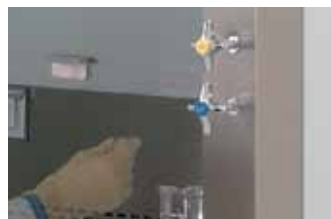
Remote Controlled Service Valves
